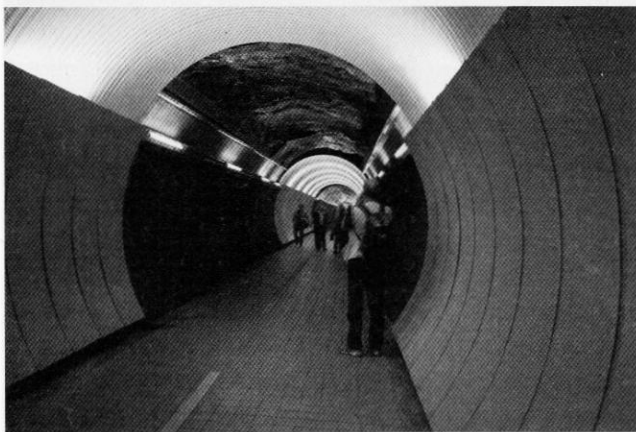
Halfway point in the Brunkebergs pedestrian and bicycle tunnel. Photo Lars Hansson
